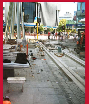
Above: Tram Tracks being laid in High Street City Mall.
