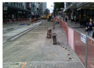
Service lane foundation in place and pedestrian ways being prepped for paving.
