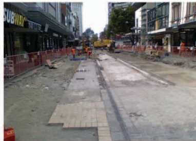
Service lane foundation in place and pedestrian ways being prepped for paving.
